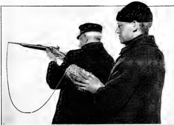
The Old 56-Caliber Sharpe's Carbine Is Also Used Now as a Line Shooter. A Blank Cartridge Is Used to Fire the Projectile to the Vessel in Distress
